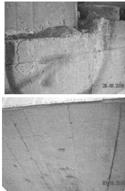
Figure A2: Typical pier of the viaducts, delaminations at an area \sim 50 \cdot 50\text{cm}^2 under the beam bearing at pier M1 and delaminations and visible reinforcement at the bottom part of the girder of pier M3
