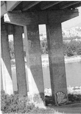
Figure A2: Typical pier of the viaducts, delaminations at an area \sim 50 \cdot 50\text{cm}^2 under the beam bearing at pier M1 and delaminations and visible reinforcement at the bottom part of the girder of pier M3
