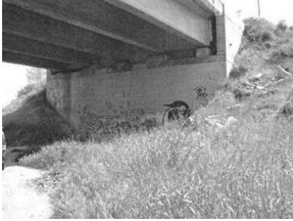
Figure A1: Abutment A0 – General view and vertical crack at the whole height
