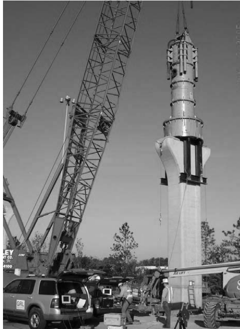
Figure 6: Hammer on Pier, Lee Roy Selmon Crosstown Expressway
