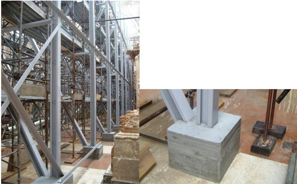
Figure 1. Built-up columns in an all FRP spatial truss structure and concrete foundation, [24], [25]
