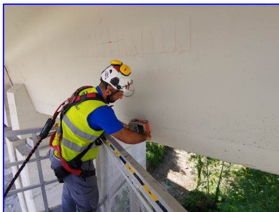
Figura 1: Georadar in quota su by bridge
