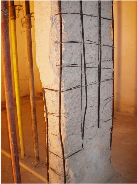
**Fig. 1** State of severely damaged corroded column
