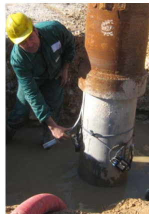
Wireless sensors on pile
