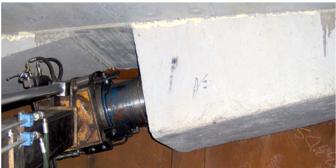
Figure 8 Precast anchorage blocks
