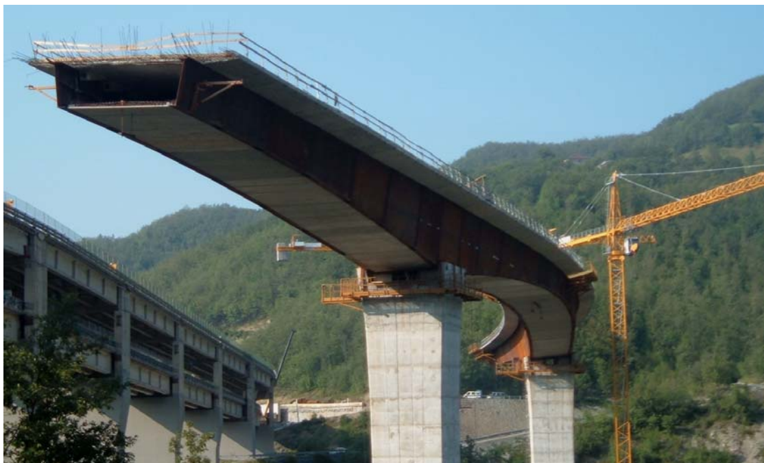
Figure 10 Completed cantilever spanning 60m
