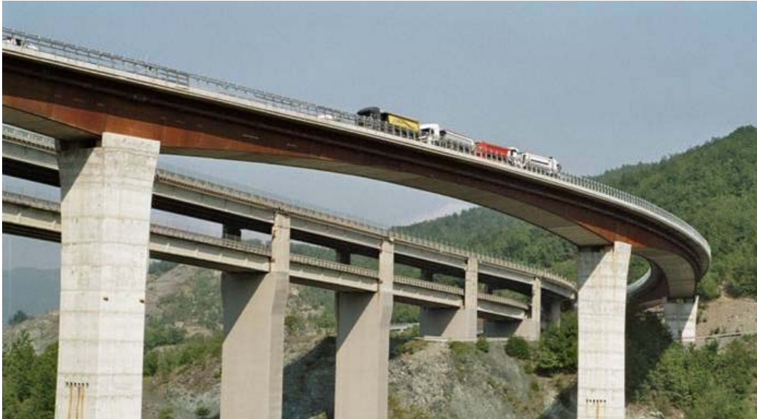
Figure 16 Completed bridge during the load test
