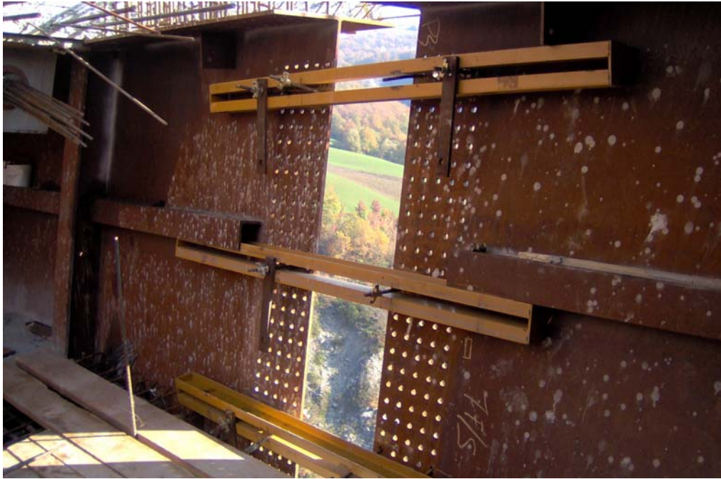
Figure 11 Final connection between adjacent cantilevers
