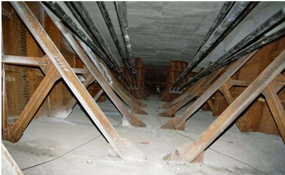
Figure 12 Internal stiffeners
