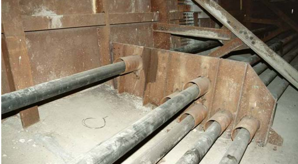
Figure 13 External tendons deviators
