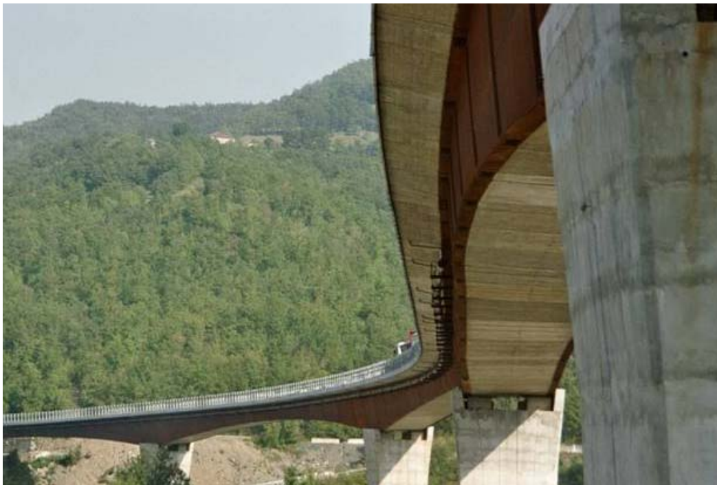
Figure 17 View of the bridge during the load test
