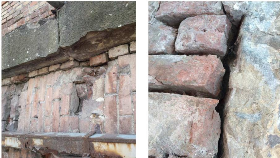
**Figure 4** – View of the damaged masonry at the drainage pipe and on a stone cornice
