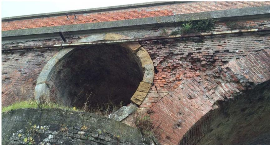
**Figure 3** – View of the masonry damage in the spandrel wall
