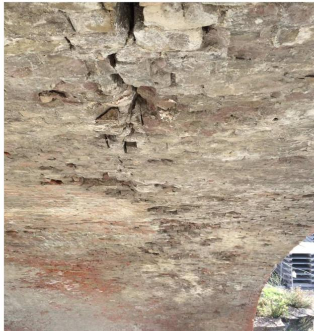
**Figure 19** – View of the masonry damage and salt spread at the arch intrados
