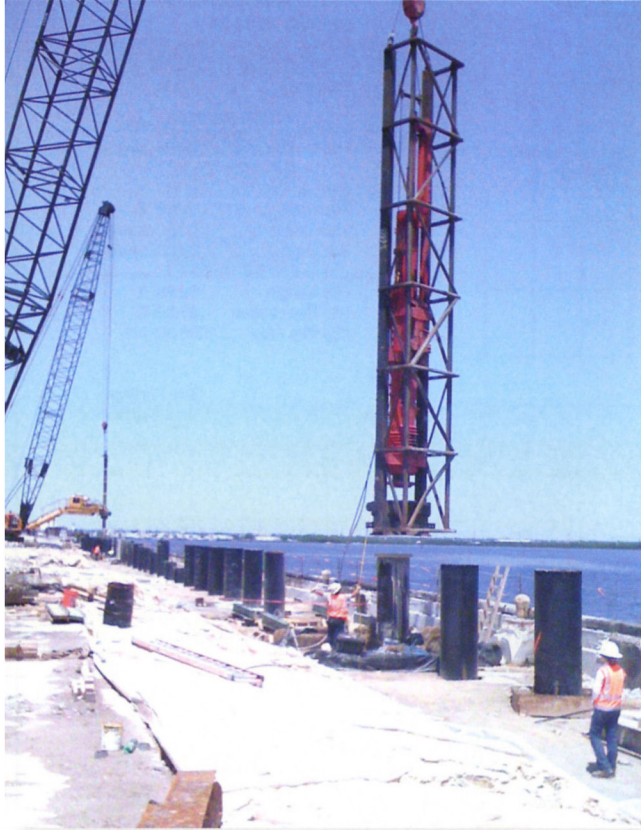
Figure 2: General view of jobsite.
