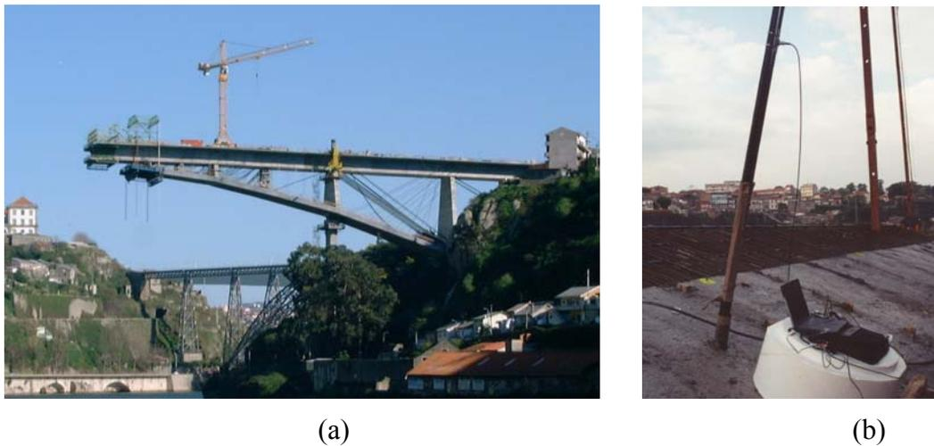
Figure 28 – (a) View of instrumented cables (b) Measurement of vibration on a suspension cable of the arch
