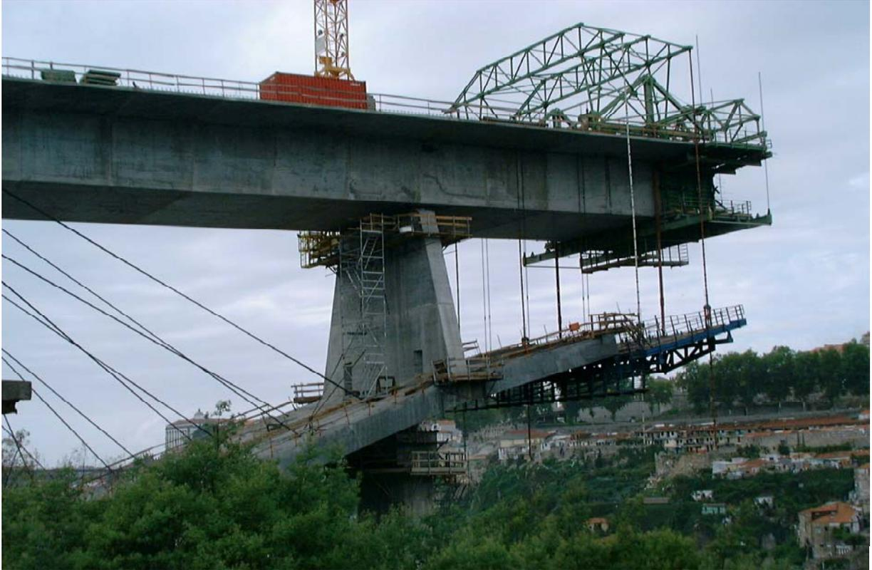
Figure 16 – Double formwork traveller
