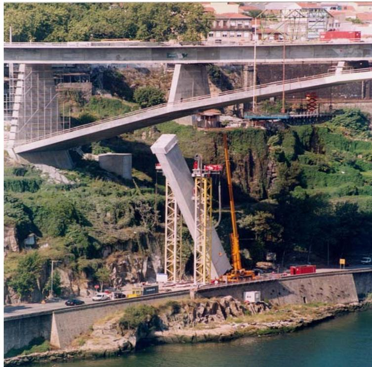
Figure 15 – Removal of the provisional pillar on the Oporto side of the river
