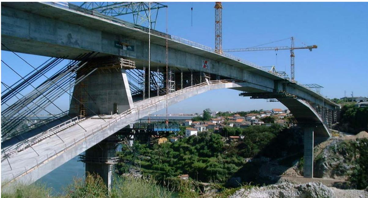
Figure 14 – General view of the bridge before provisional elements were dismantled
