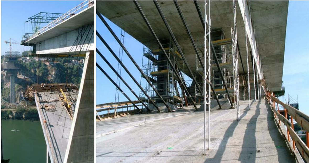
Figure 11 – Stays and suspension bars for the arch
