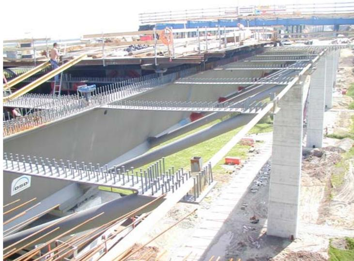
**Fig. 3.2: Valley bridge Reichenbach – open box-girder with outside compression struts and steel ties**
