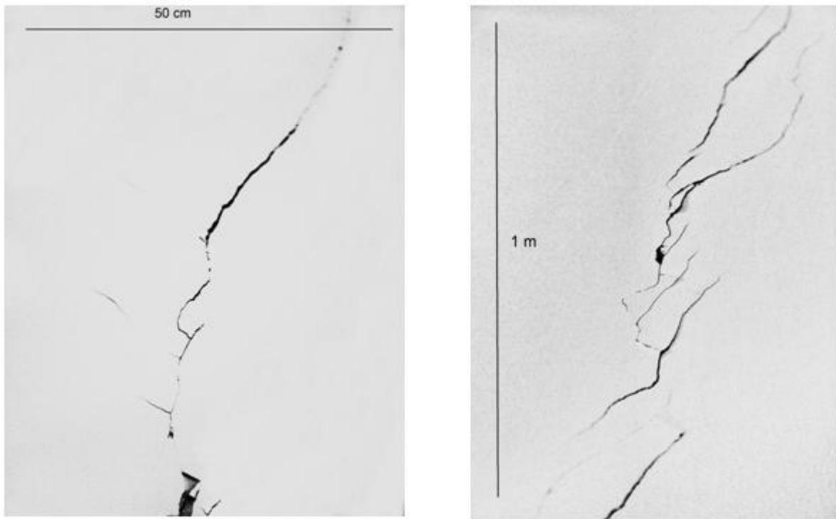
Figure 4. Example of damages (fissures) suffered from tower B as a consequence of the 20th May 2012 earthquake. The fractures have size of the order of meters [courtesy of L. Vigliotti and M. Rovere]. The most part of fractures developed on walls parallel to the transversal axis of the tower, from the 5<sup>th</sup> floor upwards.
