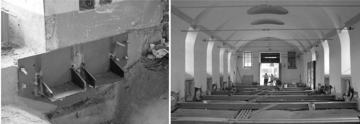
Figure 8 – Details of the intervention on Palazzo delle Carrozze in Masino Castle, Caravino (Italy): steel supports of the horizontal element (left) and overview of the intervention from above (right).
