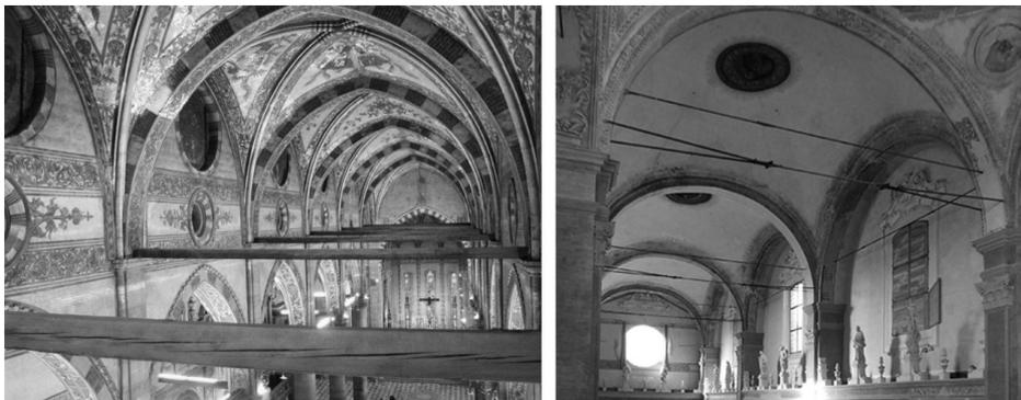
Figure 1 – View of the magnificent cross vaults of Sant’Anastasia church (Verona, Italy) with wooden chains (left) and iron chains in the central nave in San Giacomo Maggiore church (Bologna, Italy) (right).
