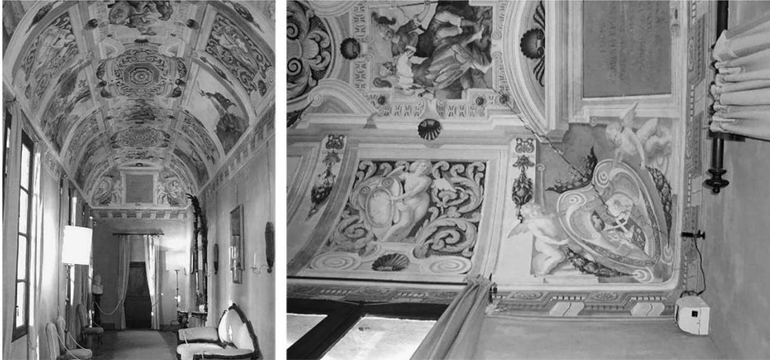
Figure 10 – Decorations at the intrados of the vault of Corridoio delle Grottesche in Castello della Manta in Manta (Cuneo, Italy). Overall view (left) and detail of a remarkable crack on the corner (right).
