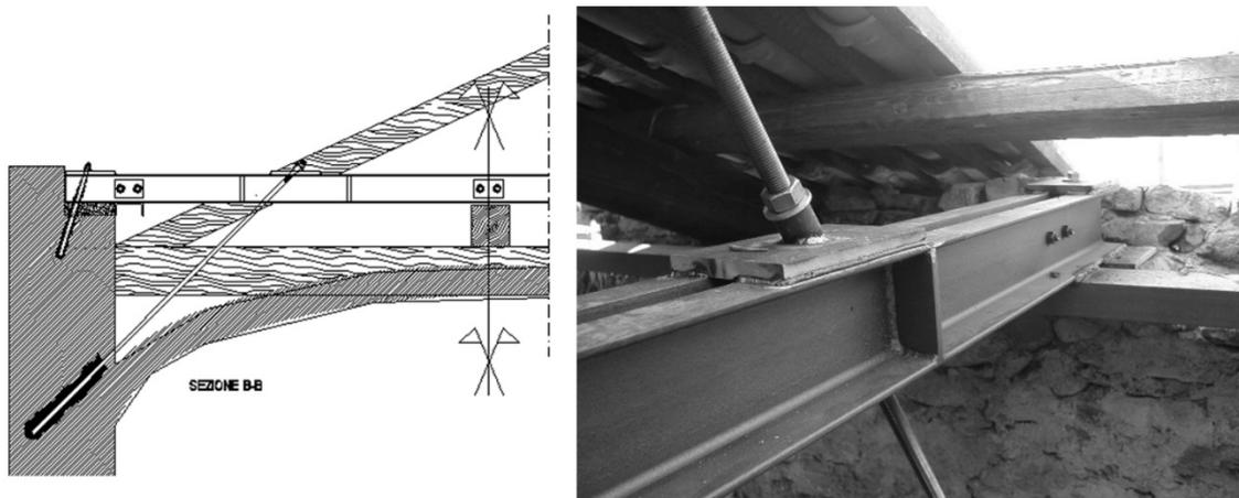
Figure 11 - Intervention with the new clamp technique on the Corridoio delle Grottesche's vault. View of half span as drafted (left) and realization (right).
