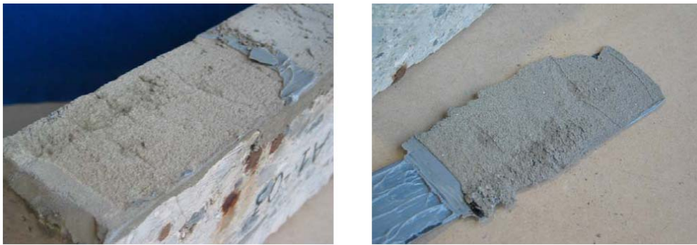
Fig. 28: Debonding by thin topping material shear failure
