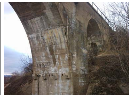
Fig. 15. Arch bridge near Hadzhi Dimovo. The lower surface has strong evidence of contamination due to water wetting.
