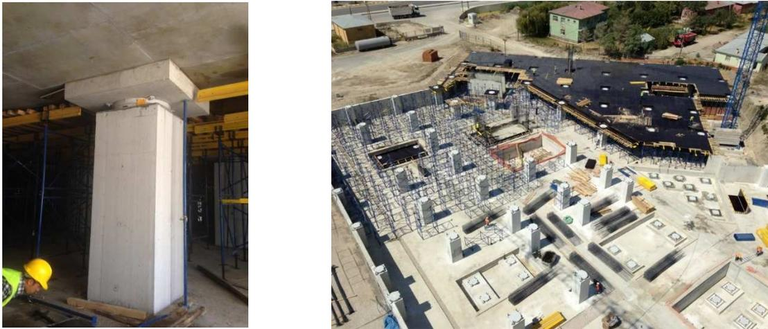
Figure 15: Van Medical Campus, Turkey - Isolation unit installed on top of a column (left), aerial view of part of the hospital during installation of isolators (right).
