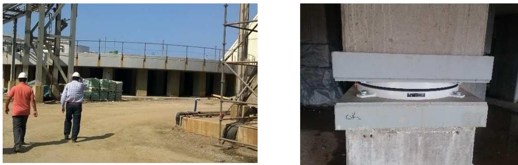
Figure 20: Ammonia storage tank in Samsun, Turkey, photos from the site: existing concrete slab and foundation before intervention (left), an isolator as installed in a column (right).
