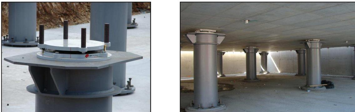
Figure 14: C.A.S.E. Project, L'Aquila, Italy - Isolation unit being installed (left), basement with installed isolation units (right).
