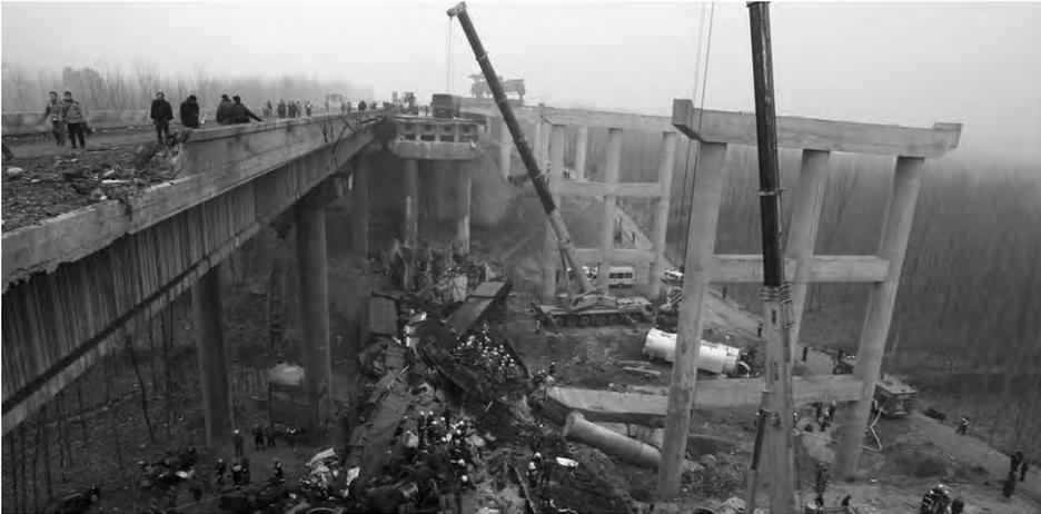
Fig. 1: Explosion on a highway bridge in China caused by a truck carrying fireworks.
