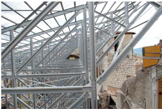
**Fig. 1.** Details of a PFRP-steel connection in the spatial structure covering the S. Maria Paganica church after the earthquake
