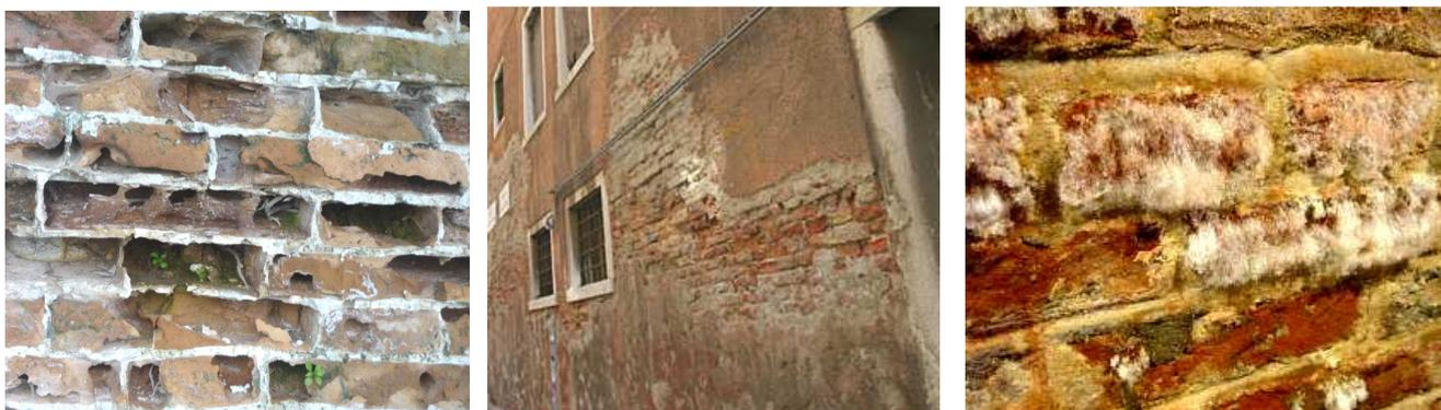
**Figure 2.** Examples masonry walls decay induced by salt weathering
