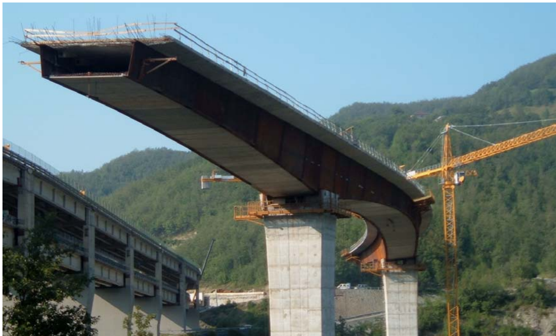
Figure 10 Completed cantilever spanning 60m
