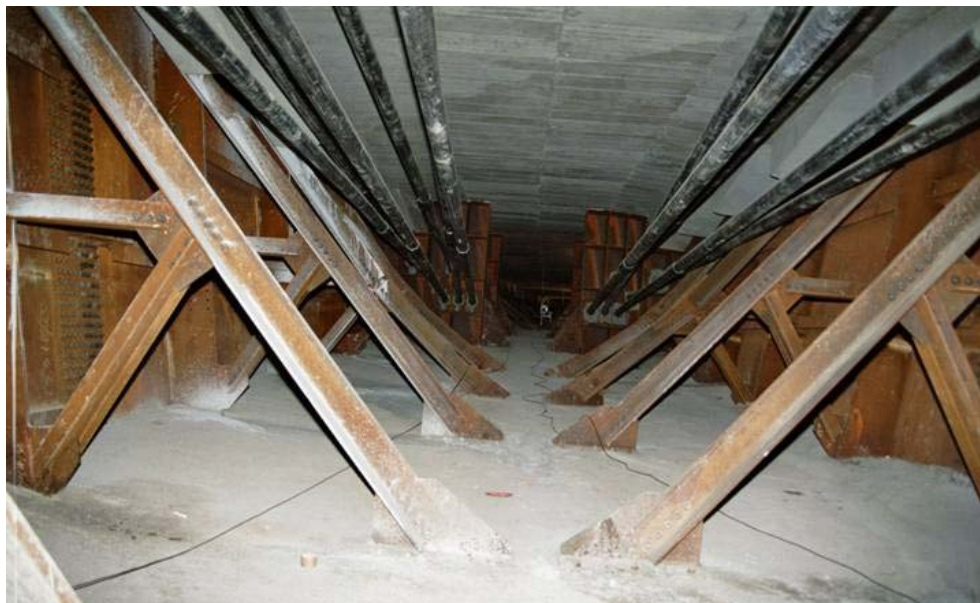
Figure 12 Internal stiffeners
