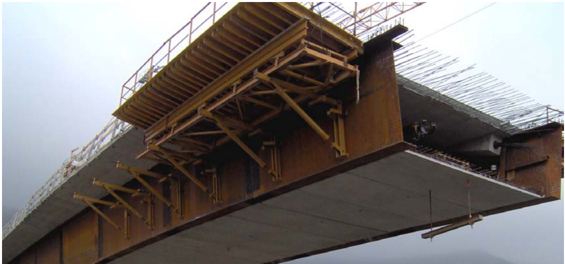
Figure 7 Bottom and top chords with formwork and scaffolding
