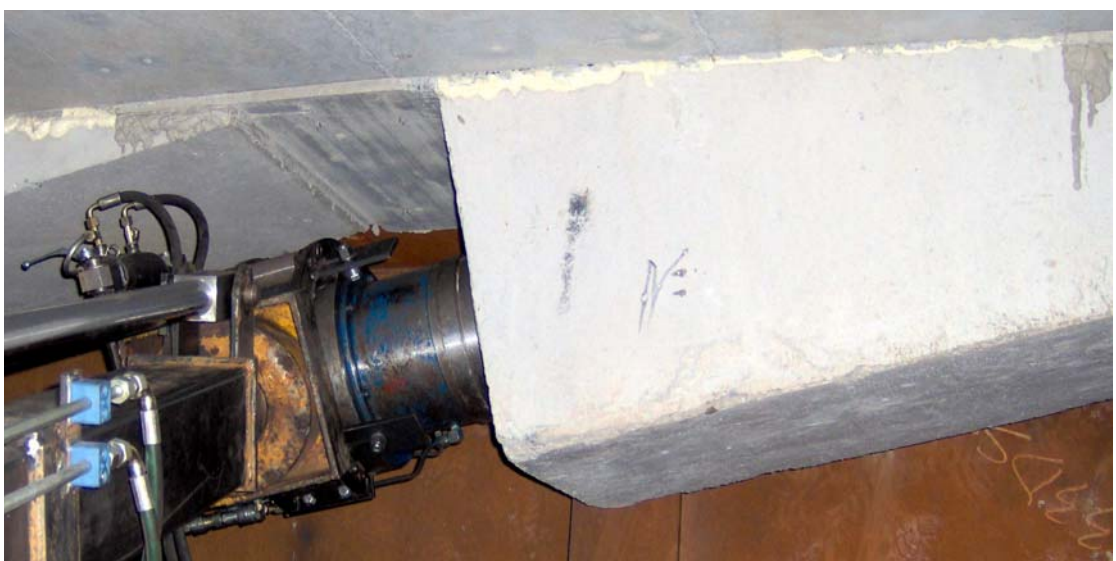
Figure 8 Precast anchorage blocks
