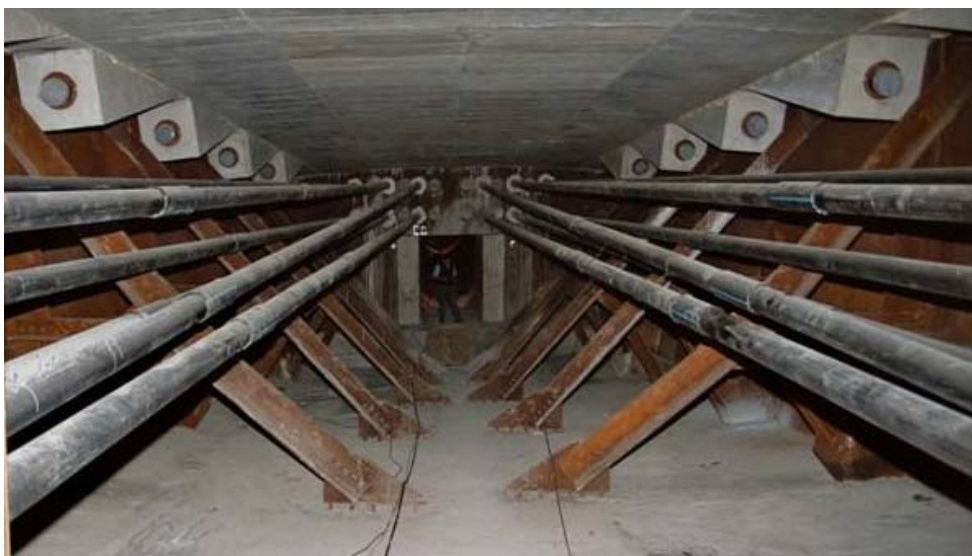
Figure 15 Internal view of external tendons near the pier segment
