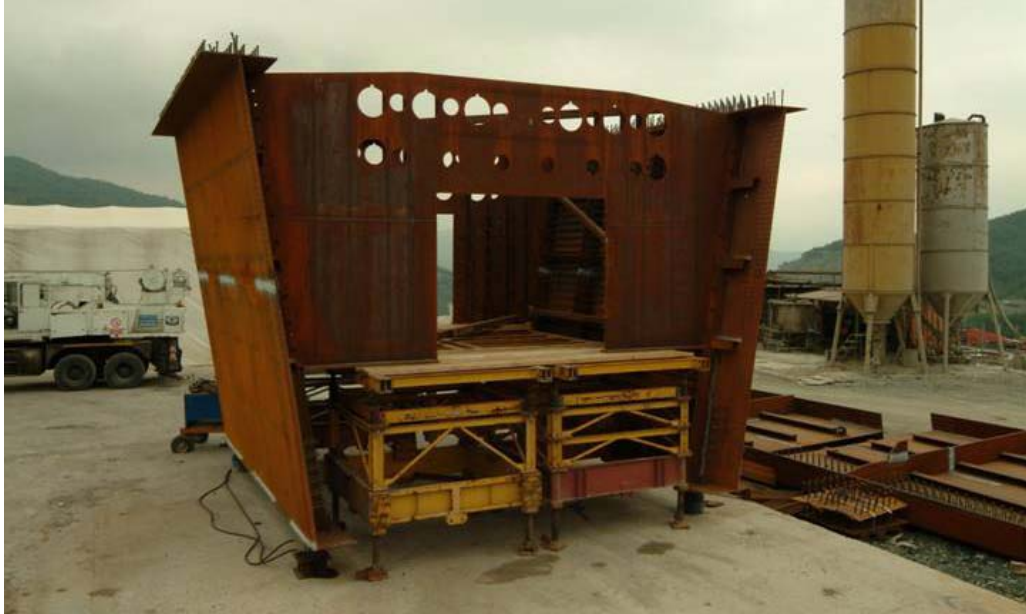
Figure 5 Pier segment ready to be assembled
