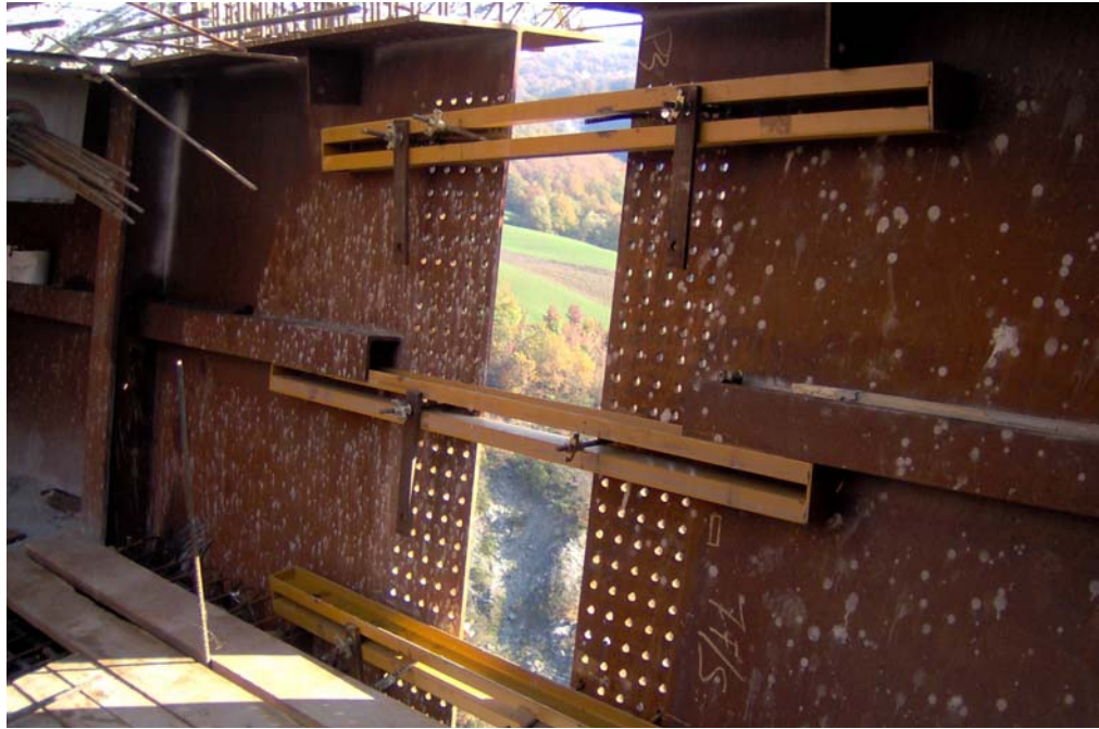
Figure 11 Final connection between adjacent cantilevers
