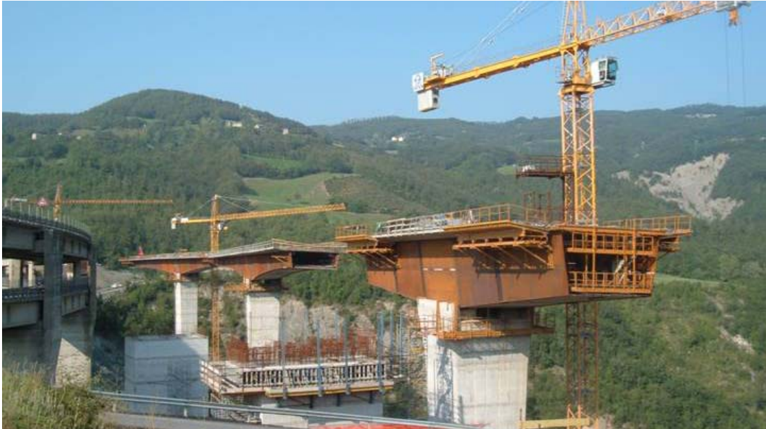
Figure 9 Parallel construction of several hammers
